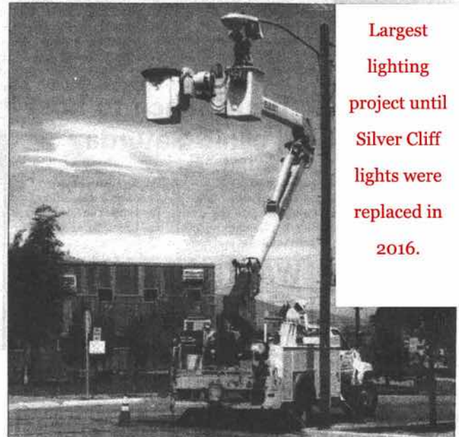
Crews with WestPlains Energy spent last week replacing the town of Westcliffe's 44 street lights with fully shielded fixtures. The new fixtures direct light to the ground where it is needed and protect the Valley's night skies. --Trib photo
